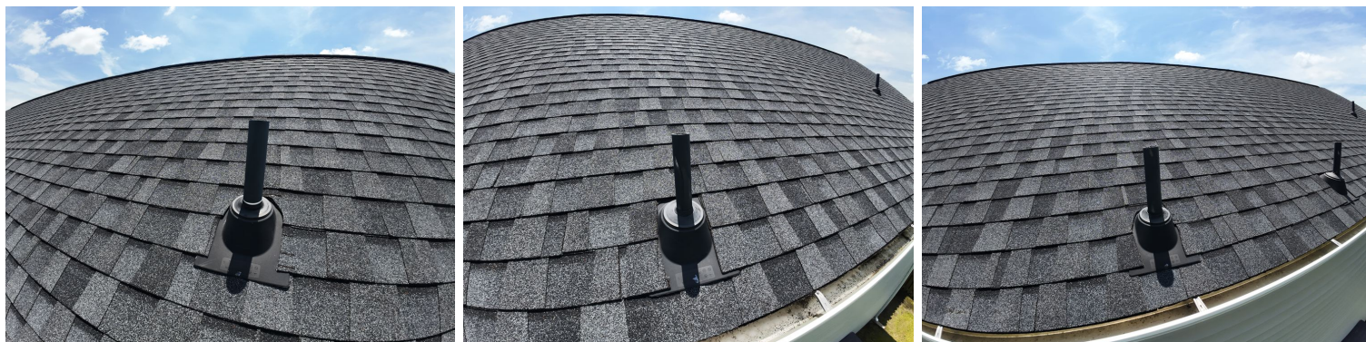
Roof penetrations and flashing
